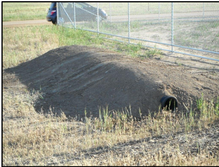
Figure 5. Artificial den for kit foxes at the Topaz Solar Farms, San Luis Obispo County, California.
