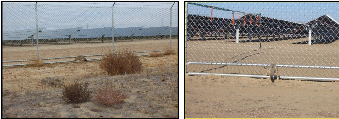
Figure 6. Security fence around solar arrays showing modifications to allow passage of kit foxes at the Topaz Solar Farms, San Luis Obispo County, California.
